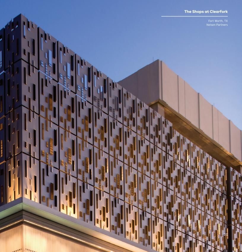
A stunning combination of functionality and aesthetics – the Perforated Panel Series provides necessary airflow and/or shade to a structure without sacrificing style or design. Virtually any shape and pattern can be perforated into the panels and used for a myriad of applications.
