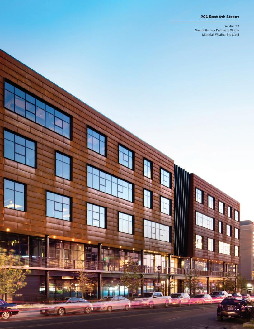
Gone are the days of flat and featureless facades. Our Shadow Series panels let you add depth and definition to any architectural design. Individual panels can be extended at varying depths to create texture or a dynamic variation in patterns, all while keeping the substrate and weather barrier in the same plane.
