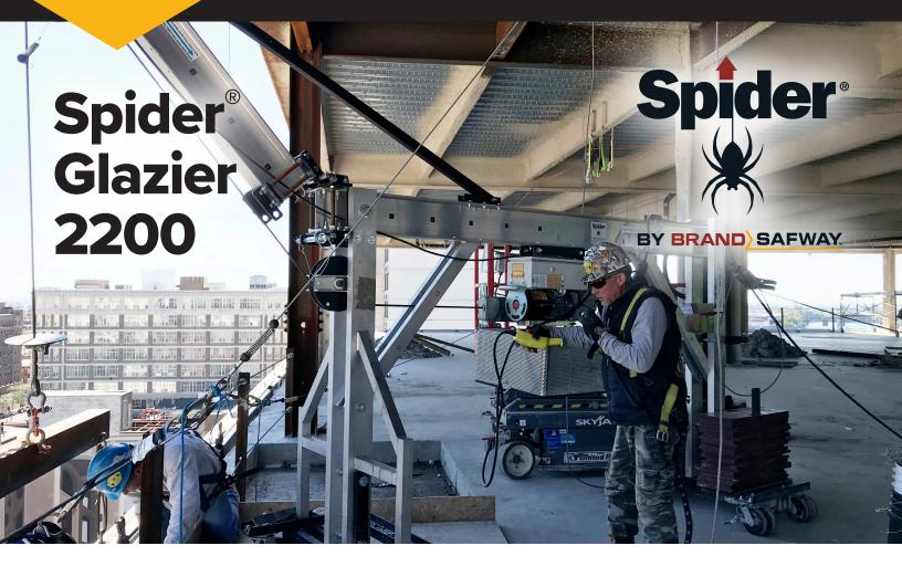
A mobile, counterweighted lifting solution for challenging curtain wall applications on high elevation job sites
