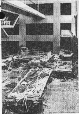
Walkway collapse in 1981 killed 114 persons.
