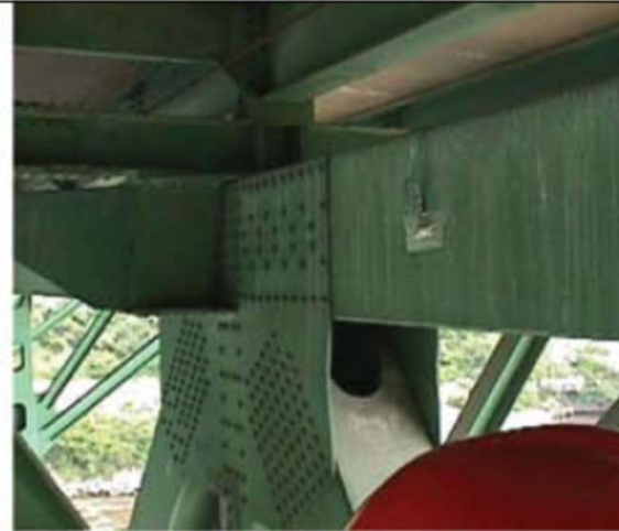
U10E looking north
